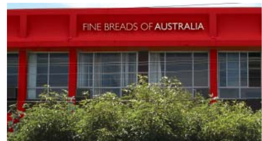
Fine Breads of Australia head office located at Brookvale.
